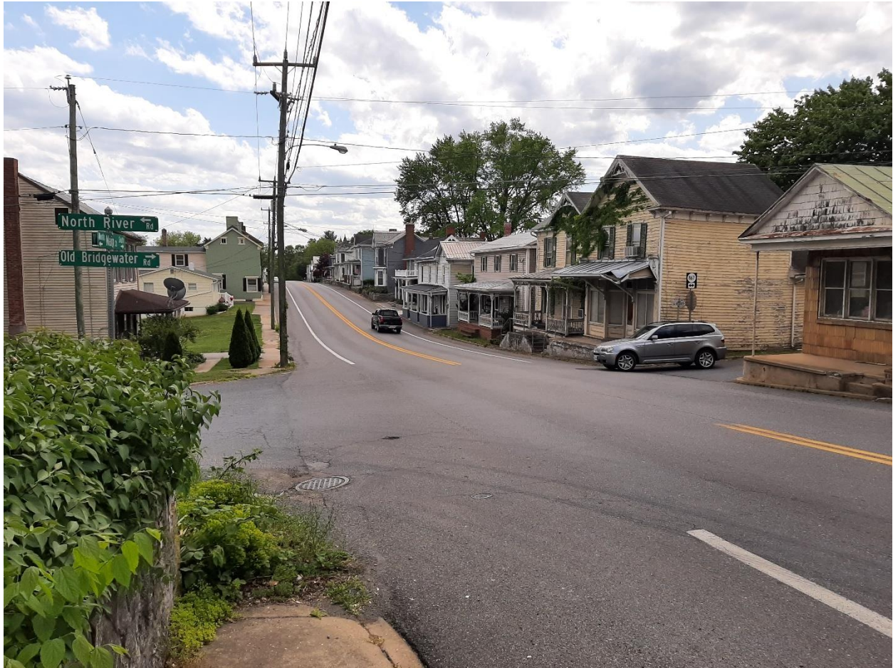
Figure 23. The streetscape at the intersection of Old Bridgewater and US 11.
