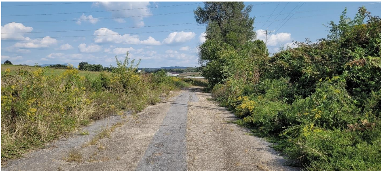
Figure 22. Looking east at an unfinished Parsons Court
